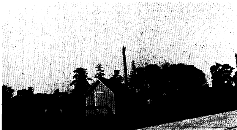
Gas purification plant of the Dominion Natural Gas Company in the Declute field.
