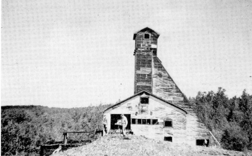
Headframe, Patterson copper property, Pacaud township.
