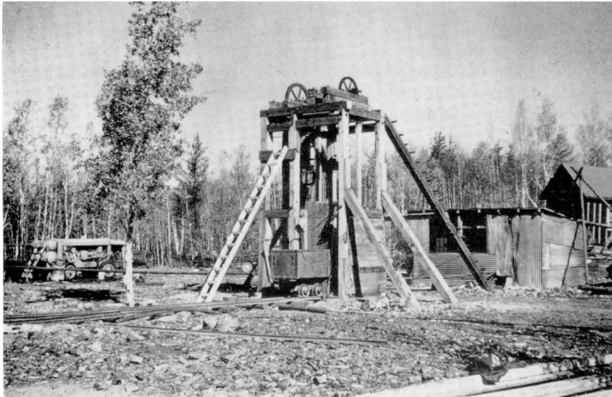
Small headframe erected in 1955 over the original Amity shaft by Mirla Exploration, Limited.
