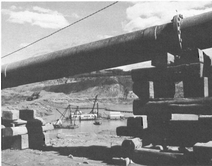
Photo 35 Dredging silt from the bottom of Steeprock "Lake". (Courtesy Ont. Dept. Tourism and Information).
