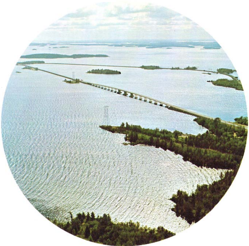
Photo 17 Aerial view of the causeway across Rainy Lake near Fort Frances. The rock fill of the embankments is made up of three rock types: syenite, hornblendite and ancient sediments. (Courtesy Ont. Dept. Tourism and Information)
