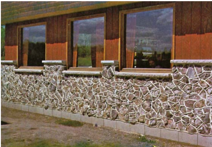
Photo 2. Decorative and durable wall facing is a popular use of amethystine rock as shown in this picture of a highway restaurant at Sibley.
