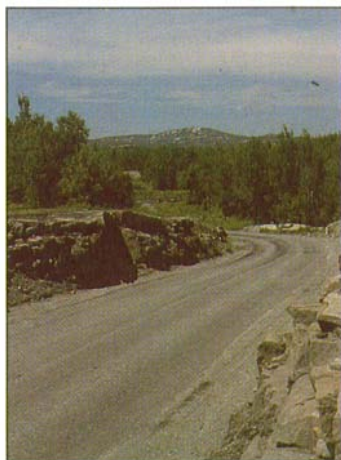
Photo 27. Roadcut in tightly folded paragneiss just east of the Bell Lake access road, 37.5 km [23.3 miles], Highway 637. Silver Peak is visible in the distance. This is the first point on Highway 637 from which any of the orthoquartzite hills may be seen.
