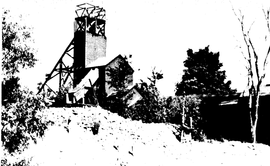
The Rogers mine, No. 1 Shaft, 1962.
