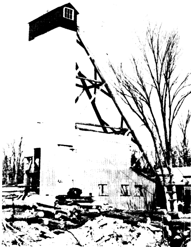
The Rogers mine, No. 4 Shaft, 1947.
