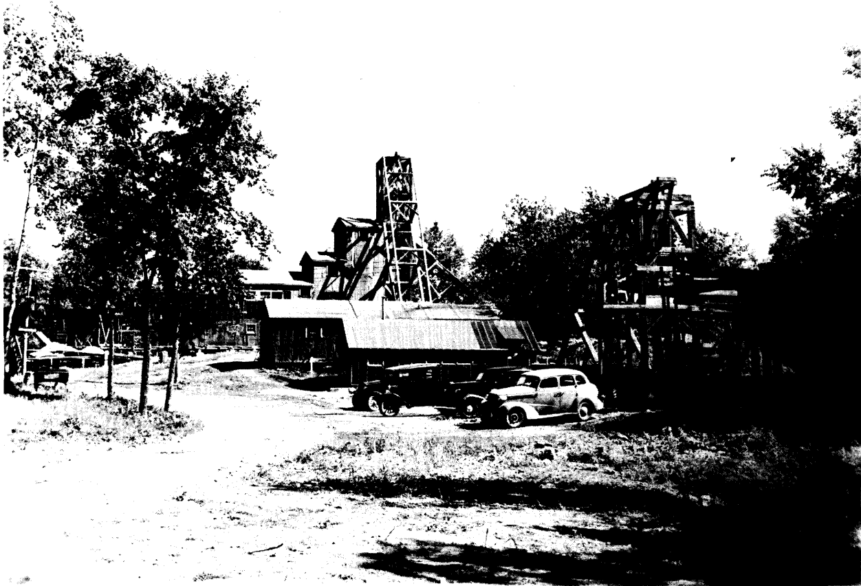
The Perry mine, 1942.
