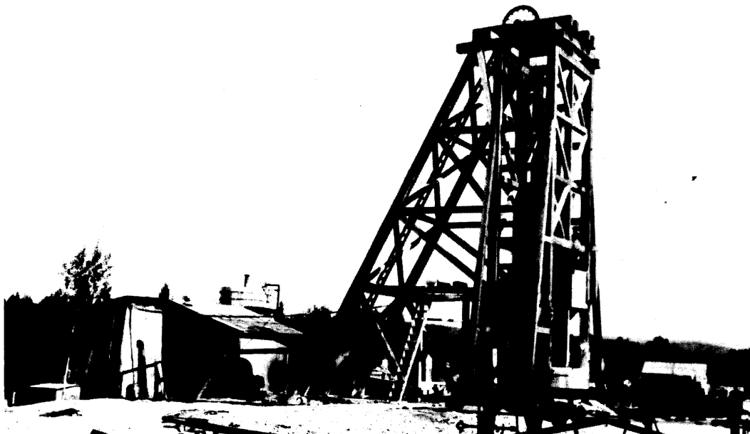
The Noyes mine, No. 2 Shaft, 1941.
