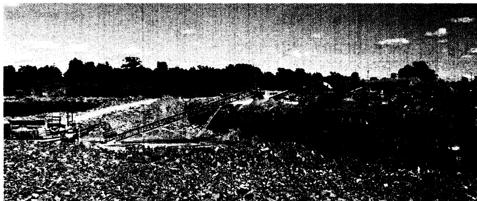
Photo BR-8-1. PRIMARY AND SECONDARY CRUSHING AND SCREENING FACILITIES AT THE LAWSON (ATHENS NO. 2) QUARRY (LOOKING NORTH).
