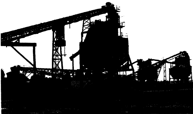
Photo CW-14-2. PROCESSING PLANT (LOOKING SOUTH); MacLEOD QUARRY.
