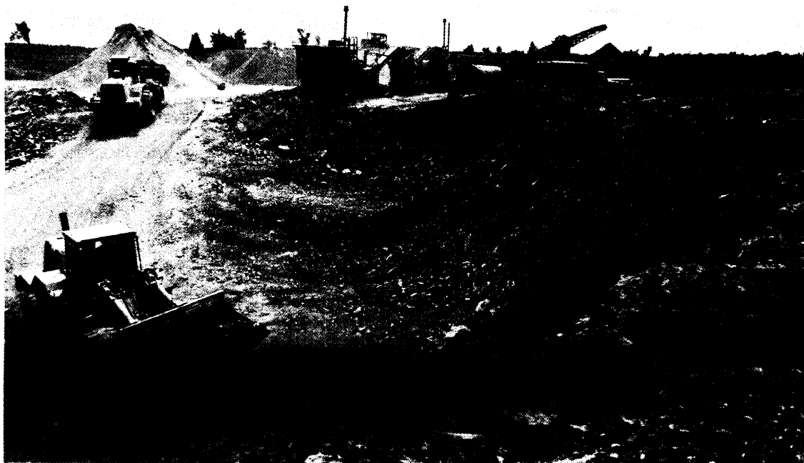
Photo CW-26-1. OPENING OF FIRST LIFT AND PORTABLE PROCESSING PLANT AT DUVAL QUARRY (LOOKING SOUTH).
