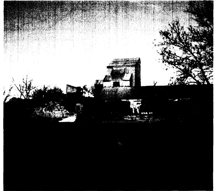
Photo TW-16-1. STOKLOSAR PROCESSING PLANT NO. 2.
