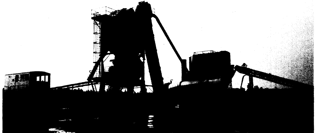
Photo CP-15-2. NEW 12,000 LB. ASPHALT BATCH PLANT AT THE MOODIE DRIVE (FALLOWFIELD) QUARRY (LOOKING NORTHWEST).
