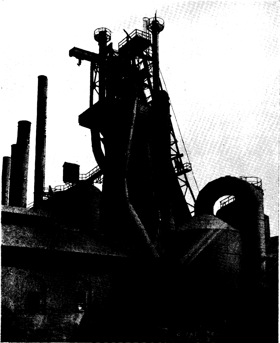
Fig. 28—"B" Furnace, Steel Company of Canada, Hamilton.
