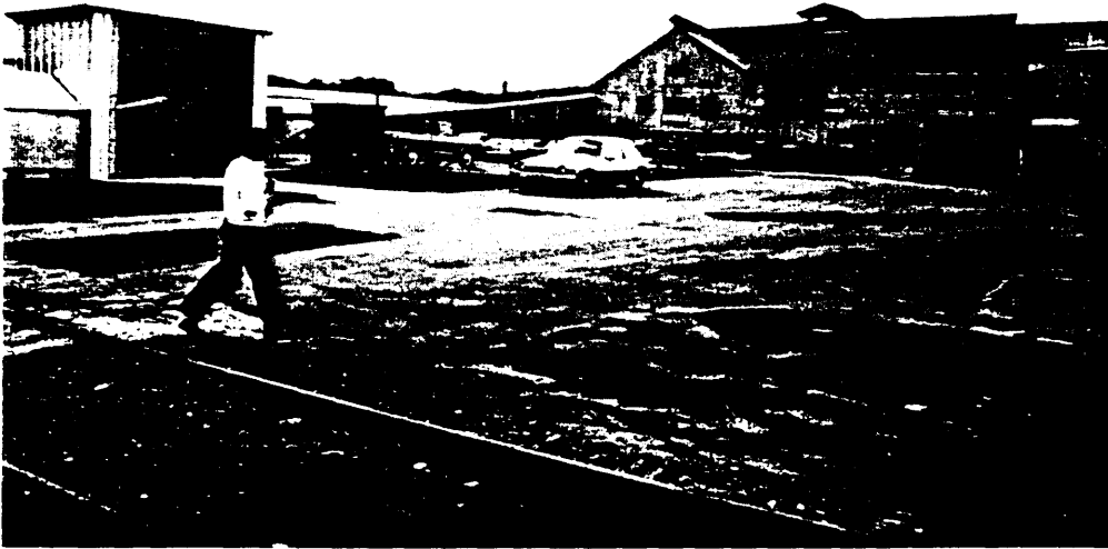
Plate 5: The rail siding and warehouse, with the old factory building in the background.
