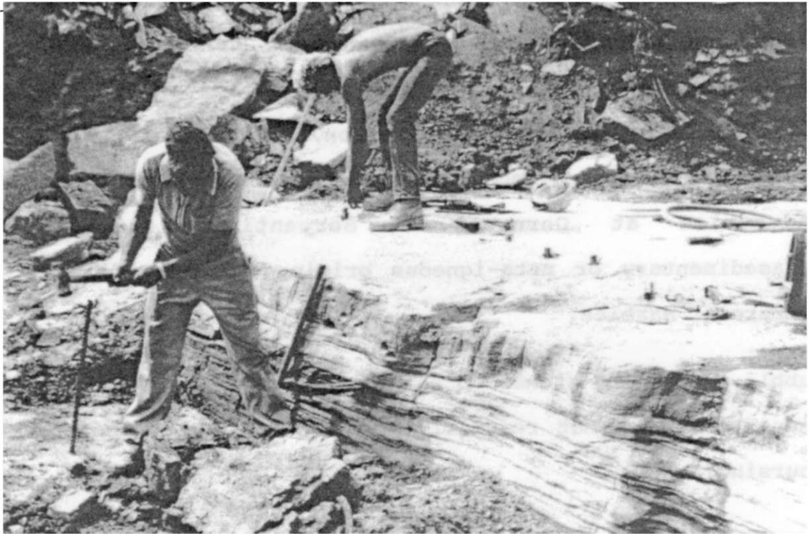
Photo 2. Plug and feather quarrying of a dolostone block, Don Ross quarry, Wiarton.
